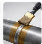
2 Priming a welded joint
